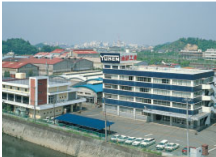
Head Office & Fujisawa Factory
